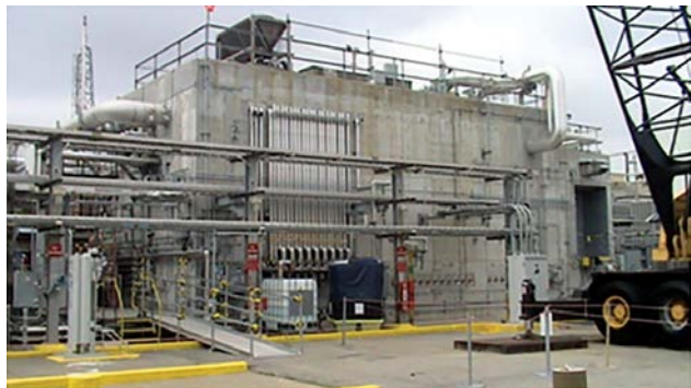
Modular unit nearing completion at the Savannah River Site for removal of radioactive cesium using the chemistry developed at Oak Ridge National Laboratory. (U.S. DOE Savannah River Site)
